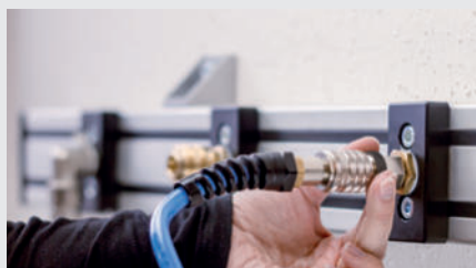
Tighten the locking nut to secure the sleeve
